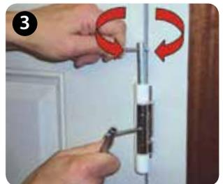
3 When in position secure the socket screw and replace the covers. **Take care not to overtighten.**
