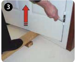
3 Lift and support the door to the required height whilst securing the socket screws. Replace the covers.
