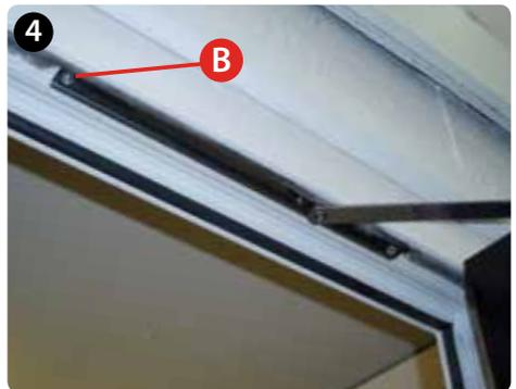
Fix frame-side of the restrictor to the outer frame using the remaining fixing screws at points B & C.
