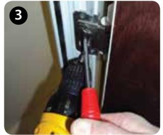
3 Secure the screws in the side plate.
