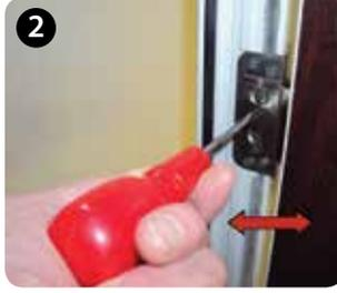
2 Lever the slide plate (B) with a screwdriver in the adjustment slot
